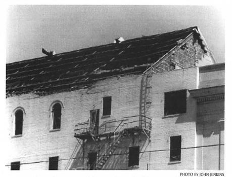
Damage to the southeast corner of the Journal Record Building. Note deformation of heavy steel purlins disposed horizontally across the roof, over the rafters.
